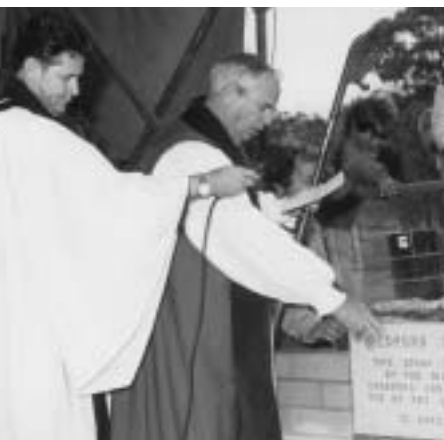
Bishop Warren laying the Foundation Stone.
